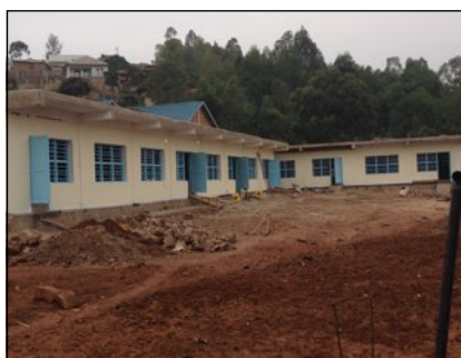
The new classrooms
